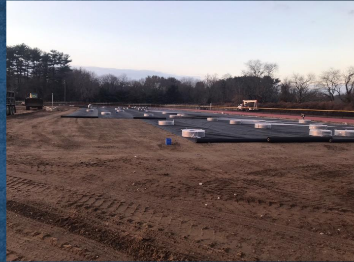
Installation of Geotextile drainage fabric with ADS drainage system
