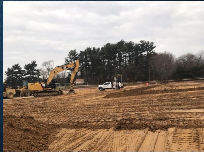
Graded subgrade material
