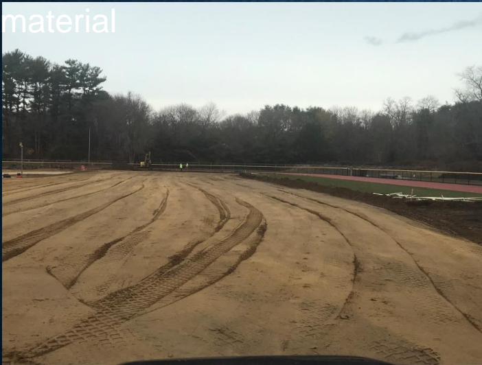
Graded subgrade material
