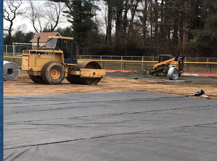
Geotextile drainage fabric installation
