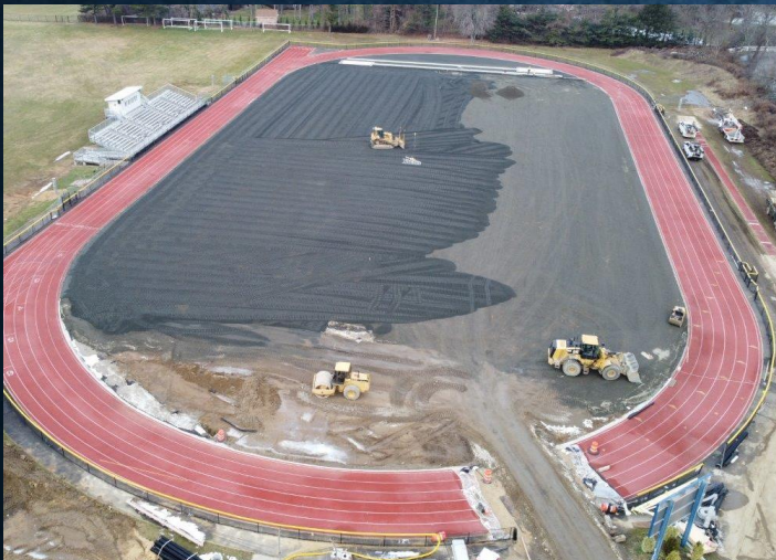
Aerial Pictures of blue stone screenings being applied to the field
