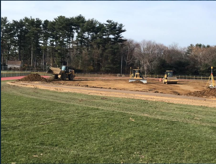
Beginning removal of top organic material
