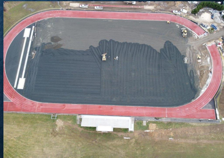
Aerial Pictures of blue stone screenings being applied to the field
