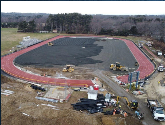
Aerial Pictures of blue stone screenings being applied to the field
