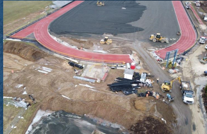
Aerial Pictures of blue stone screenings being applied to the field
